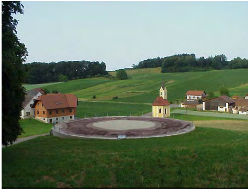
Photograph 6.7: Closed storage tank of digested material (concrete cover)
