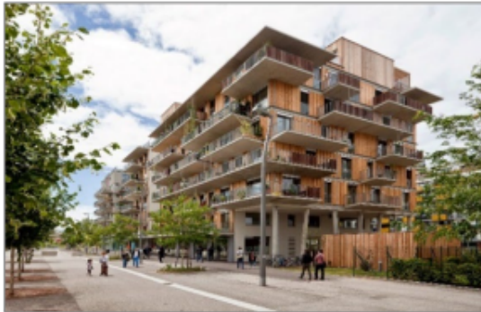
Fig.1 EXTERIOR VIEW, WEST VIEW, RESIDENTIAL PROJECT VIENNA
